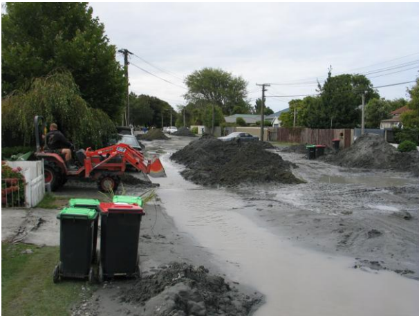
Figure 18: Piles of liquefaction ejecta cleaned from residential properties and roads, ready for removal by heavy earth moving machinery at Bracken Street in the suburb of Avonside. (Photo credit: Jarg Pettinga).
