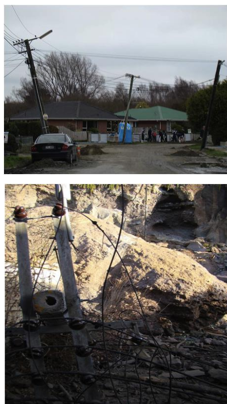
Figure 10: Orion 11 kV faulted cables following 22nd February Earthquake liquefaction maps from Tonkin and Taylor (2011) and Cubrinovski and Taylor (2011).
