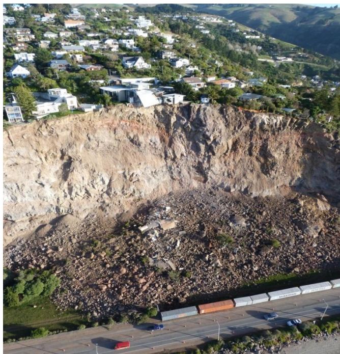
Figure 3: Cliff collapse at Clifton Hill following the 22 February and 13 June 2011 earthquakes - flown 14 June 2011. Note the partially collapsed house and use of ballasted shipping containers as temporary catch fences (Photo credit: Marlène Villeneuve/David Bell).
