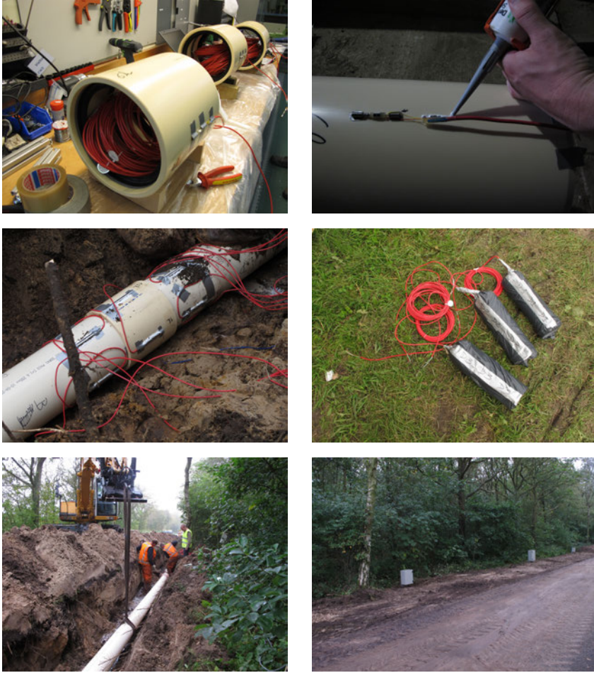
Figure 4.2: Photos taken during the installation of the sensors. Top left: the strain gauges fixed on the joints. Top right: a strain gauge being fixed on a pipe. Middle left: the dummy strain gauges inside sealed PVC canisters. Middle right: the installation of the pipe. Bottom left: the strain gauges fixed to a joint and two pipes. Bottom right: following the installation, the three cabinets are visible above ground.
