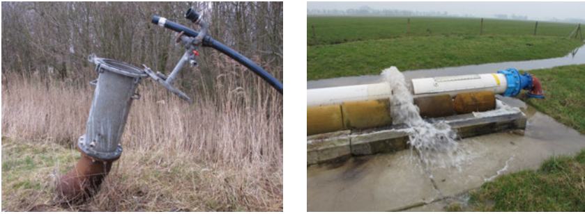
Figure 3.11: Entry point with flange and hose (left). Exit point with sliding door above ground level (right).
