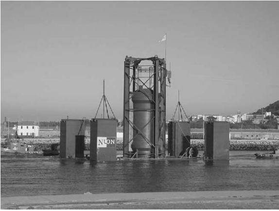
Fig. 2. Photo of the AWS pilot plant before submerging.
