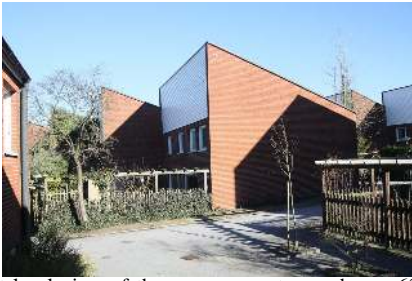
Fig. 3. Street level view of the measurement area, house 63, in which the receive antenna array was positioned.
