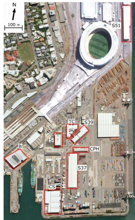
Figure 24: CentrePort Wellington map showing buildings surveyed (Base image from Google Earth™).
