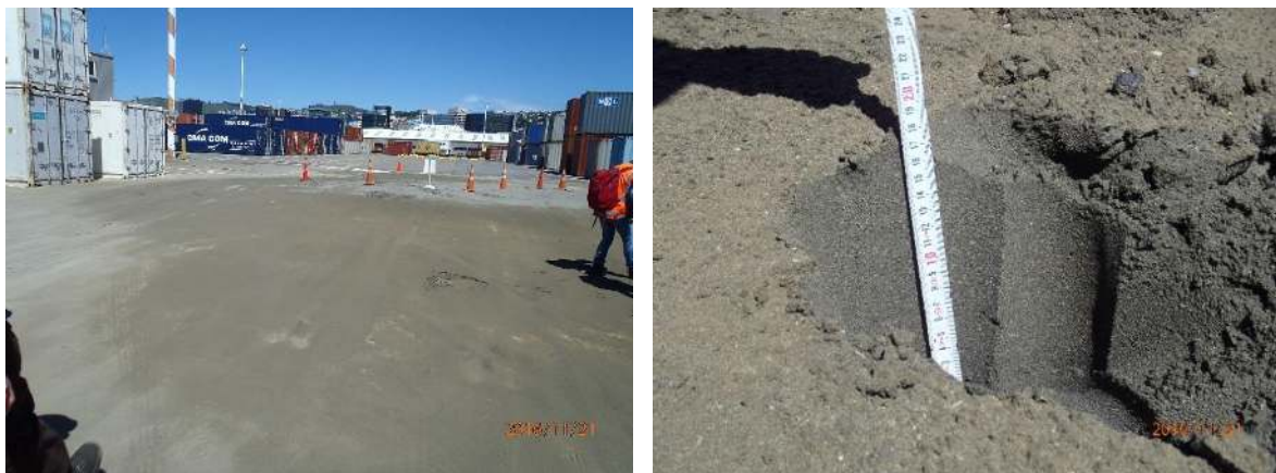
Figure 10: Sandy liquefaction ejecta with trace gravel among area of 1970's end-dumped quarry rock reclamation (i.e., Thorndon Reclamation) at STA 145 and approximately 60 m west of the bulkhead. The ejecta deposit was approximately 170 mm thick at this location. Samples S11 and S12 were collected here (S41.279067° E174.788792°, taken on 21NOV2016).
