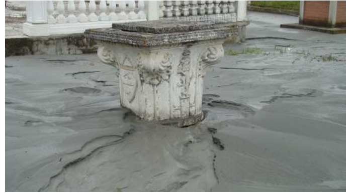
Figure 2. Example of sand ejection from a large-diameter water well at the base of the levee associated with an abandoned reach of the Reno River (San Carlo-Sant'Agostino road).
