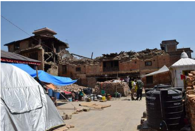
Fig. 13 Structure damage observed at Bungmati village near Bhainsepati—no evidence of liquefaction (Liq. ID 8 in Table 6) [Photo: RM Pokhrel]
