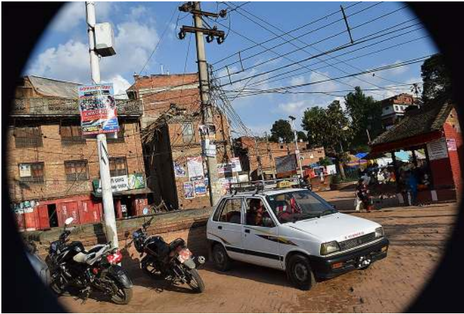
Fig. 14 Structure damage observed at Jagati—no evidence of liquefaction (Liq. ID 9 in Table 6) [Photo: RM Pokhrel]
