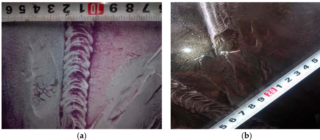
Figure 6. Inspections for external defects of pipeline girth weld: (a) dye penetrant; (b) magnetic particle.
