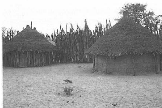
Figure 23. Two types of hut walls: wooden poles (left) and mudblocks (right). Photo: Antti Erkkilä 15.10.1996.
