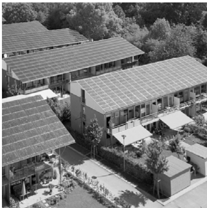
Fig. 1. Monitored Net Plus Energy Settlement, Freiburg, Germany [2]
