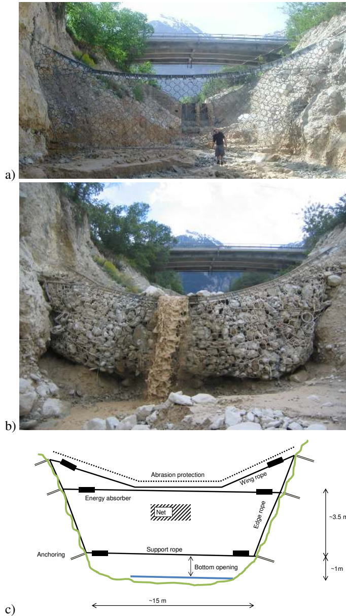
Fig. 1. a) Flexible debris flow barrier in Illgraben torrent (Switzerland); b) Flexible debris flow barrier in Illgraben torrent (Switzerland after debris flow event from 18 May 2006); c) possible arrangement of structural components of a flexible debris flow barrier (Volkwein, 2014) and its rough dimensions in Illgraben torrent.
