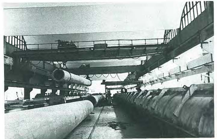
Fig. 84. Freshly cast prestressed hollow cylinder piles.
