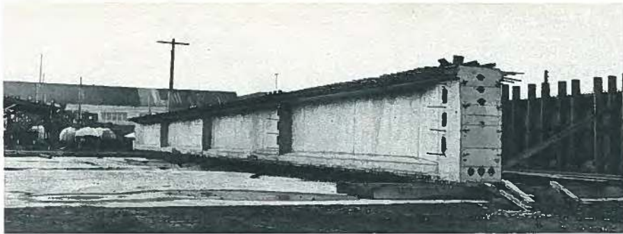
Fig. 77. Completed girder after stripping side forms.
