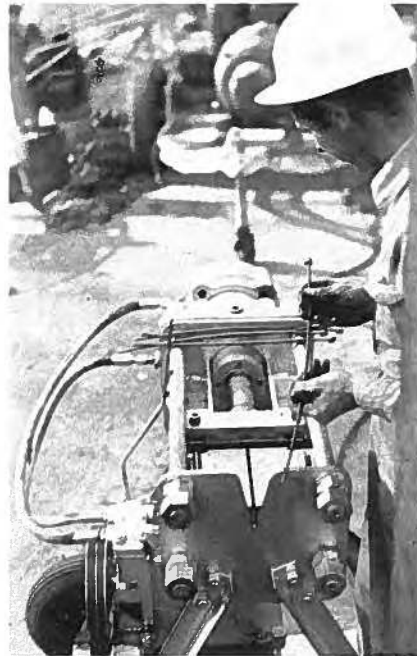
Fig. 6. Headed wire and heading machine.
