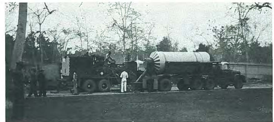
Fig. 11. Halliburton grouting the girders.
