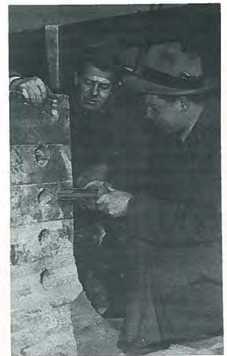
Fig. 49. The author (right) and his brother Thomas Anderson checking concrete strength of abutment with Schmidt test hammer (1951).
