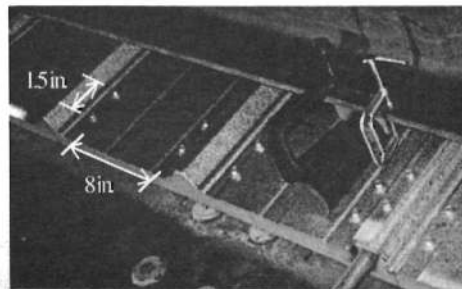
Figure 13 Selected standard panel-to-purlin and panel-to-panel fastener configuration (C-section)
