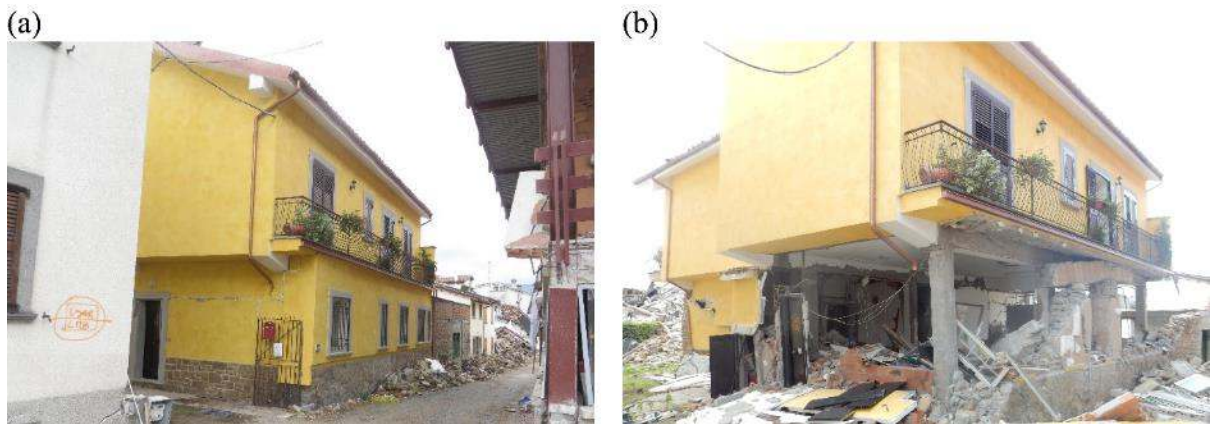
452 Figure 15. Irregular in plan reinforced concrete residential building. (a) limited damage after the 24 453 August earthquake and (b) considerable non-structural damage at ground level, failure of the infill 454 panels and residual drift.
