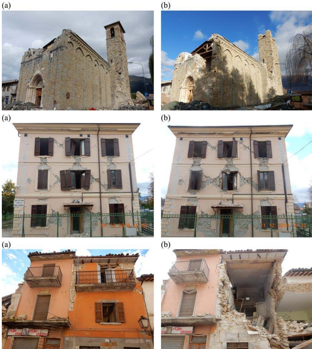
475 Figure 17. Incremental structural damage of the church of Sant’Agostino (top), the local police 476 station (middle) and one of the several masonry buildings collapsed after (a) the event of 24 August 477 earthquake and (b) the entire sequence.
