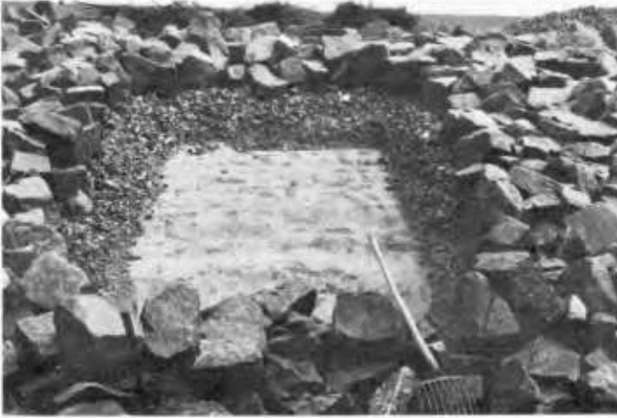
Fig. 8 Non-woven fabric after removing the cover layers
