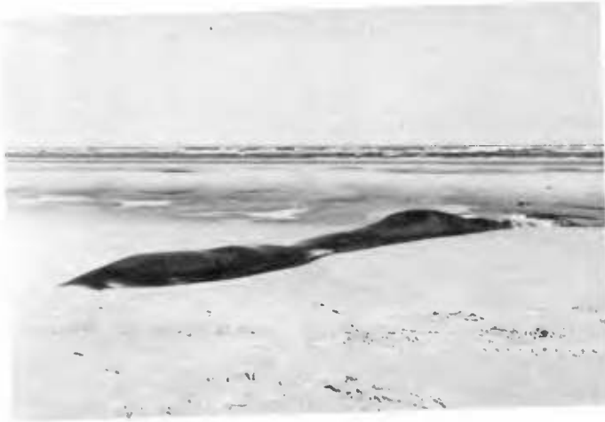
Fig. 10 Sand filled tube in a beach feeding area
