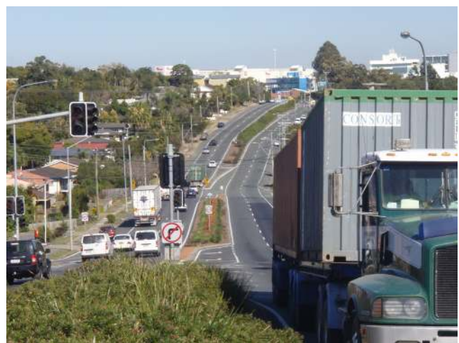
FIG. 1. (Color online) A short section of the 11 km urban corridor where the roadway is a two-way four-lane roadway with a median strip. The corridor carries some 40 000 to 50 000 vehicles per day, with up to 15% heavy vehicles. Note the residential dwellings in proximity to the roadway on the left of the photograph—typical of much of the corridor.
