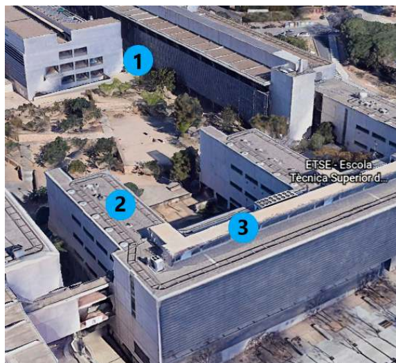
Figure 8. Location of the (1) gateway and (2–3) nodes in the second configuration. Gateway was placed at an office behind the metallic wall appearing in point 1 at ground level, while nodes were located at offices at points 2 (115 m from the gateway) and 3 (130 m from the gateway) in the third floor. Image taken from Google Earth.
