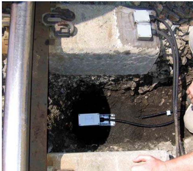
Figure 6-8: Placement of sensors between the ties at the ballast-subgrade interface.
