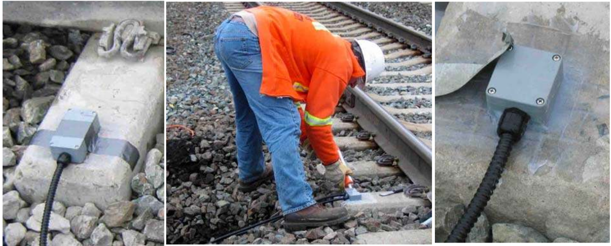
Figure 6-4: a) the epoxy was allowed to harden during the 10 minutes setting time, b) application of silicone spray to protect weathering of epoxy, c) final working stage of the sensor.
