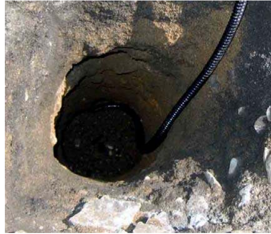
Figure 6-7: Backfilling the piezometer with Insitu soil filling.
