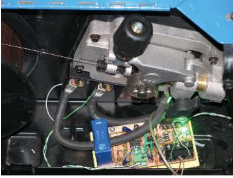
FIGURE 4: Circuit installed in welder.
