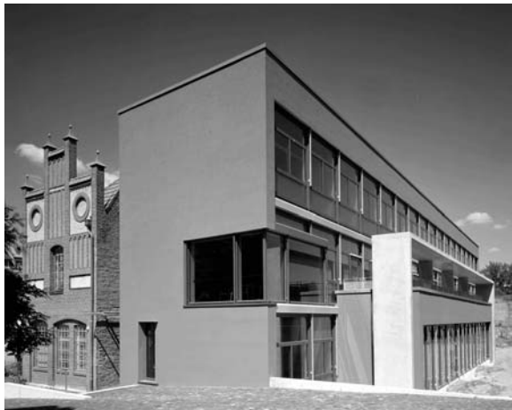
Figure 3: The office building of the Centre for Sustainable Building equipped with embedded pipes in concrete slabs as the heating and cooling system and a ground heat exchange to collect ground coolness.
