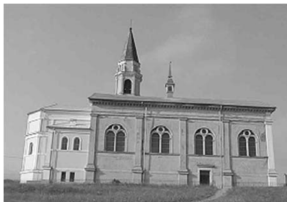
Figure 4: St. Martin church in Teharje with frescos is equipped with a wall temperisation system.
