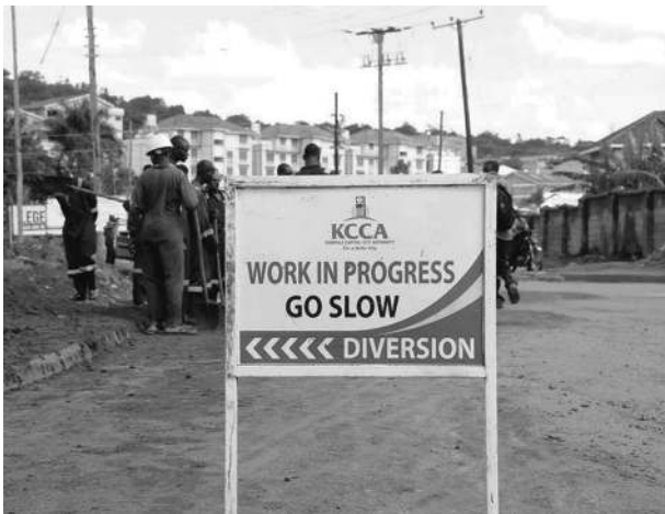
Figure 1. “Work in Progress,” posted November 18, 2014, by the Kampala Capital City Authority (KCCA). A color version of this figure is available online.
