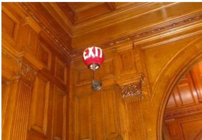
Figure 1.13: An example of the custom-made exit signs at Craigdarroch Castle (Victoria, BC) (Photo by author, 17 May 2013).
