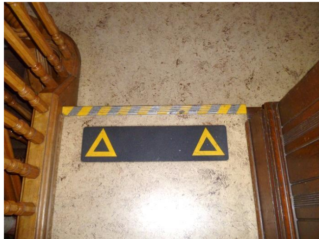
Figure 1.17: Caution tape and triangles indicating a step at Craigdarroch Castle (Photo by author, 17 May 2013).
