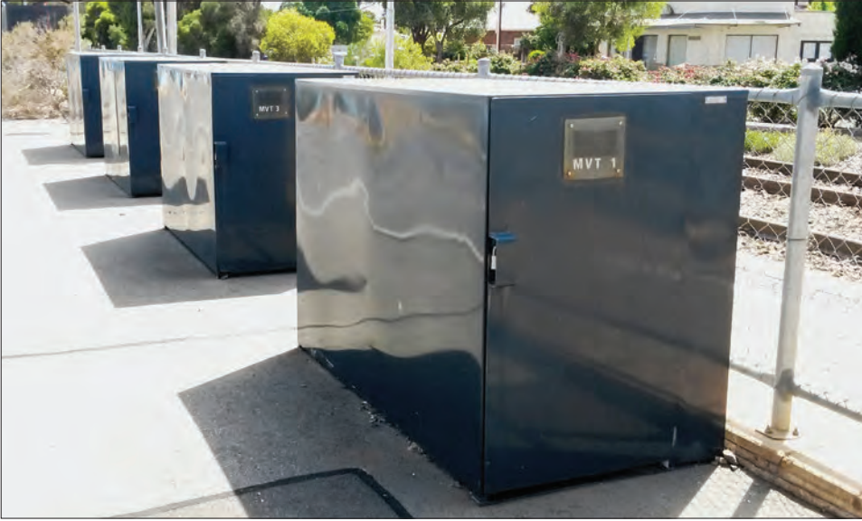
Figure 16.18: Australian Standard Class 1 locker. (Source: author's own work.)
