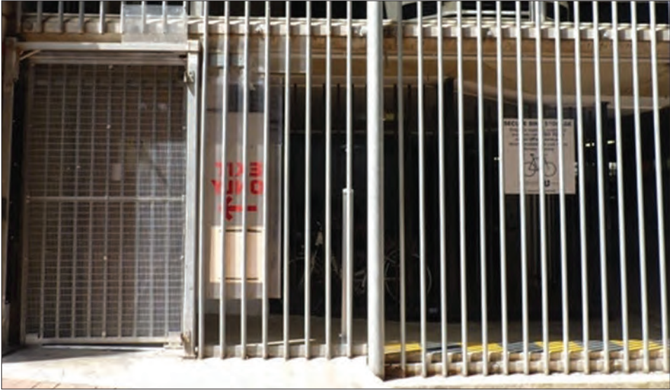
Figure 16.34: Cage parking located inside an enclosed car park, with no directional signage. (Source: author's own work.)
