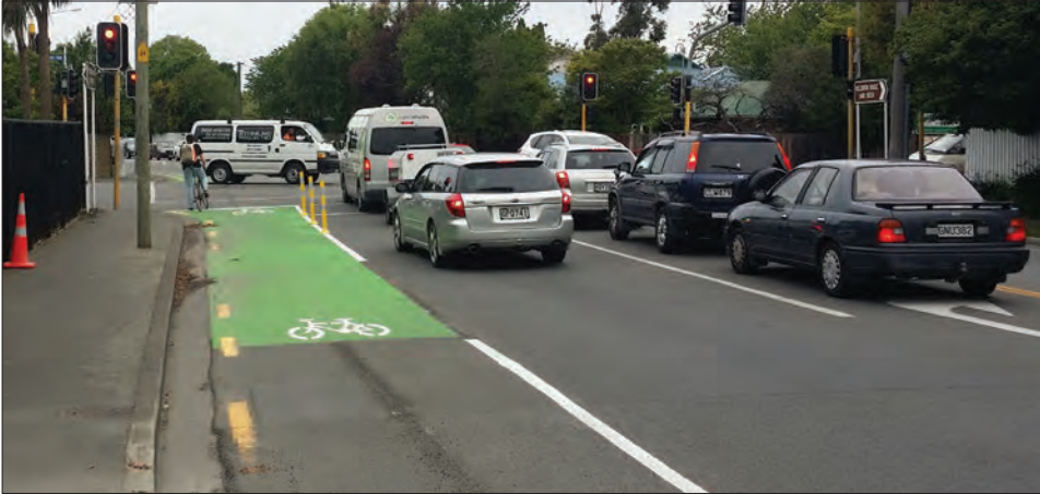
Figure 12.5: Cycle lane with separator posts and coloured surfacing in Christchurch, New Zealand. (Source: Author.)
