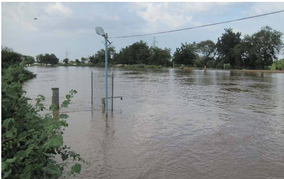
Figure 4.2: Gezira main canal at Sennar October 2011. Water is pushed up so high that the water gauge can not be read anymore.
