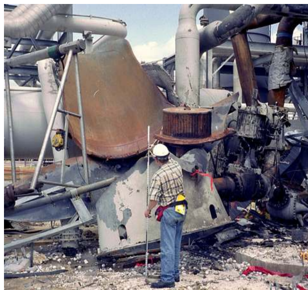
Fig. 3 Brittle fracture of a pressure vessel is sudden and catastrophic, resulting in loss of containment of product and energetic fragmentation
