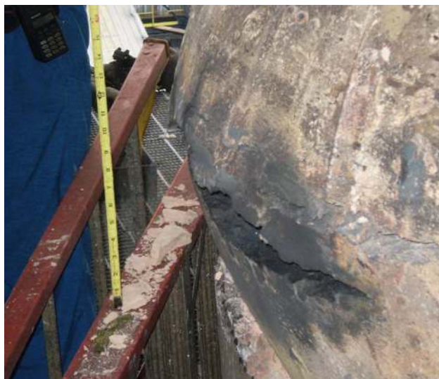
Fig. 5 Ductile fracture in a 112-mm (4.4-inch)-thick steel pressure vessel shell indicated by extensive bulging and deformation that preceded the fracture
