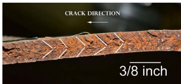
Fig. 6 V-shaped chevron marks found on a pressure vessel brittle fracture surface indicating the direction of crack propagation
