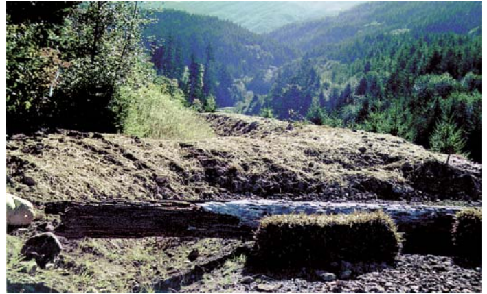
This road has been ripped and seeded, and access blocked with logs.
