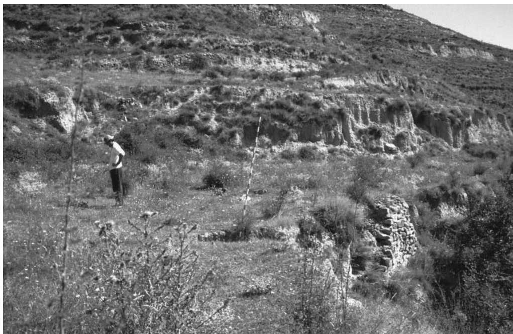
FIGURE 4 Erosion and spread of scrub on high terraces abandoned since the 1940s or 1950s. The 20–25° slope is concave. The terraces are located at a considerable distance from the village of Terroba, Leza Valley. (Photo by L. Ortigosa)
