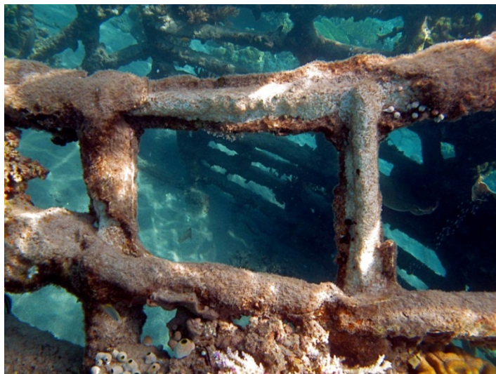
Figure 4. Self repair of Biorock damaged by big boat impact. Time series photographs by Rani Morrow-Wuigk. This structure was installed in June 2000. Note there is no rust on the steel after nearly 11 years in seawater.
