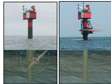
Fig. 7. Hybrid illustration of the Seaflow turbine [© MCT].
