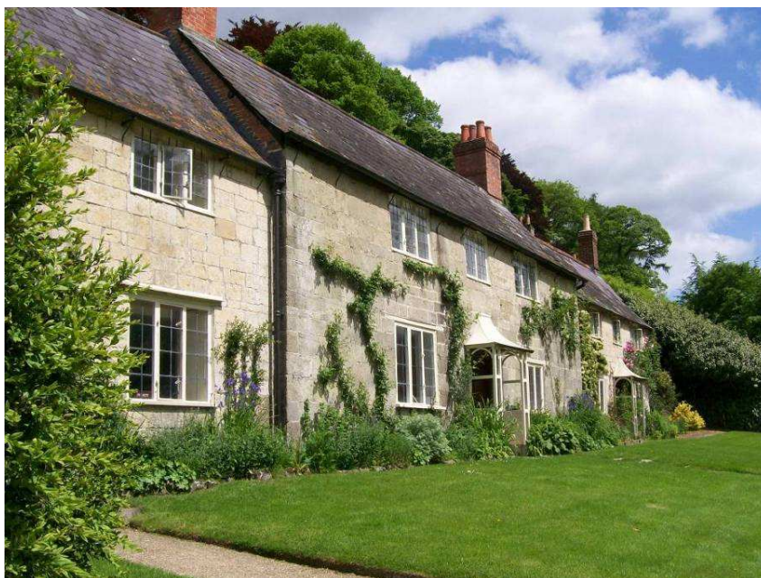
Figure 2-7: Well maintained labourers' cottages in Stourton
