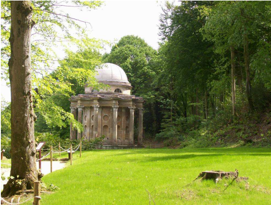
Figure 4-9: Temple of Apollo, one of the follies erected in Stourton in 1765 with a great deal of labour Source: Cathy Day
