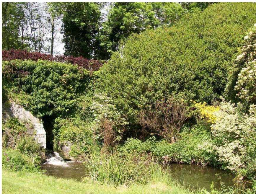
Figure 5-32 : River Stour at Gasper Mill
