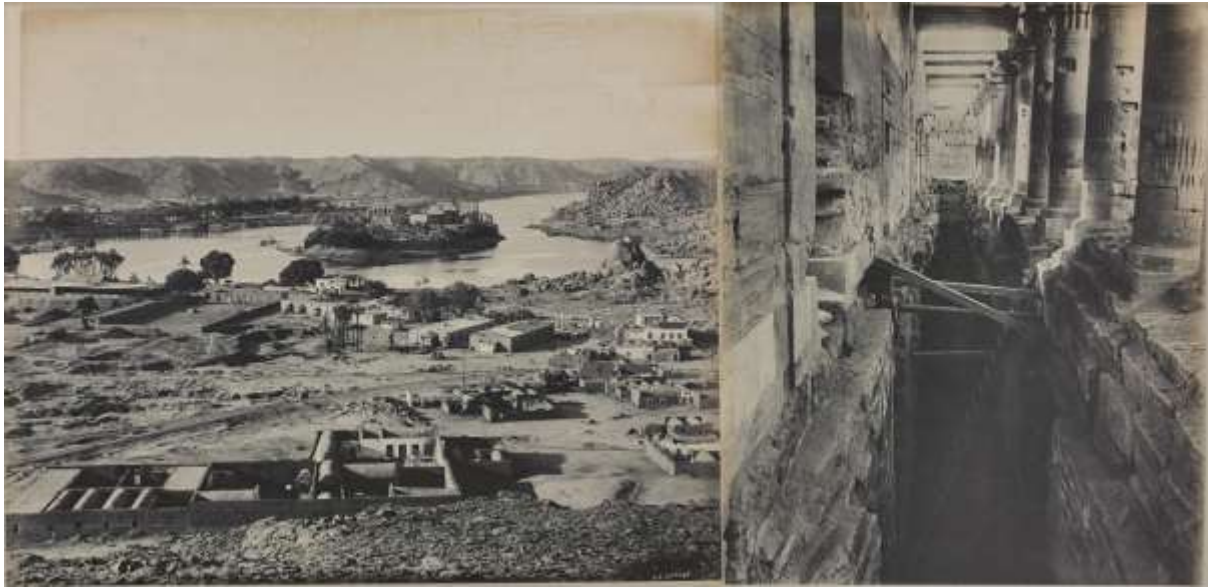
Figure 5 Left: "Island of Philae: general view." HIL 455/26. Right: "Island of Philae: View of underpinning at the Eastern Colonnade." HIL 455/27.
