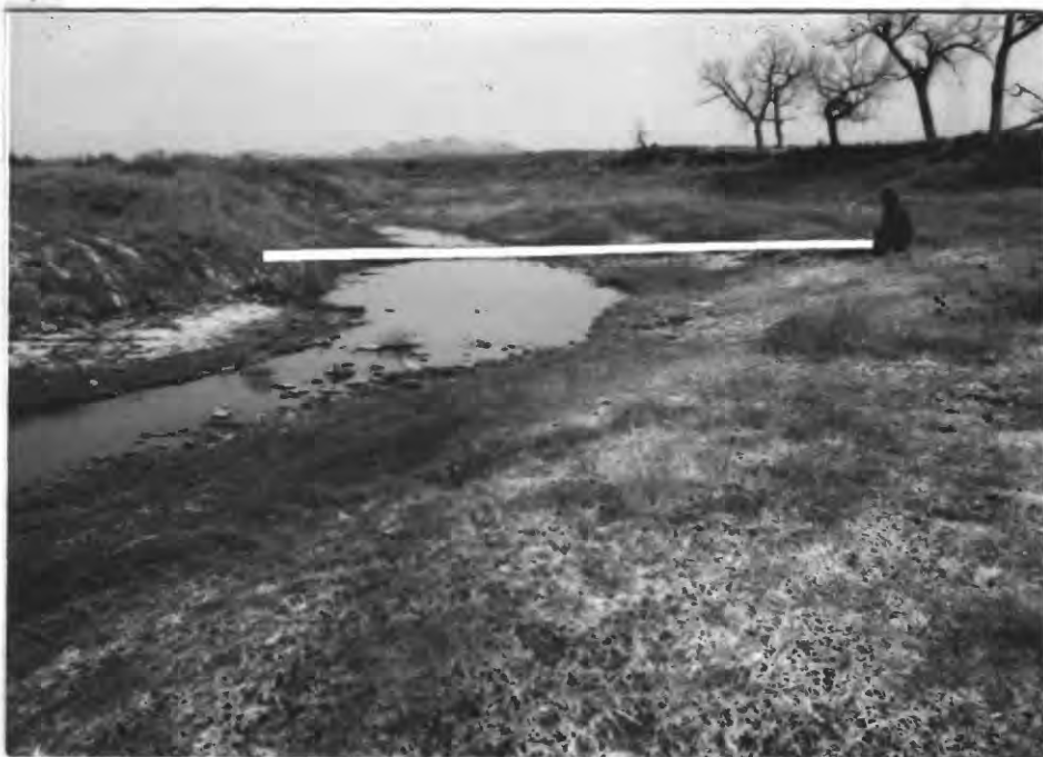
Figure 8.--Bankfull section on Pearson Creek near Decker, Montana. Section is defined by change in slope; width is about 4 feet. Site is near station 1. View is upstream.
