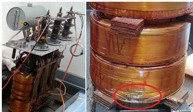
Fig. 2. A distribution transformer 22 / 0.4 kV under the test in HV laboratory with a defect in the A phase.
