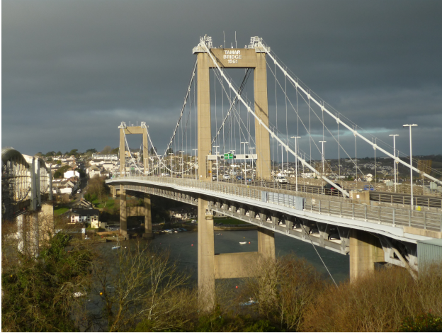
Figure 1. The Tamar Suspension Bridge in the U.K., crossing the River Tamar between Plymouth to the east and Saltash to the west.
