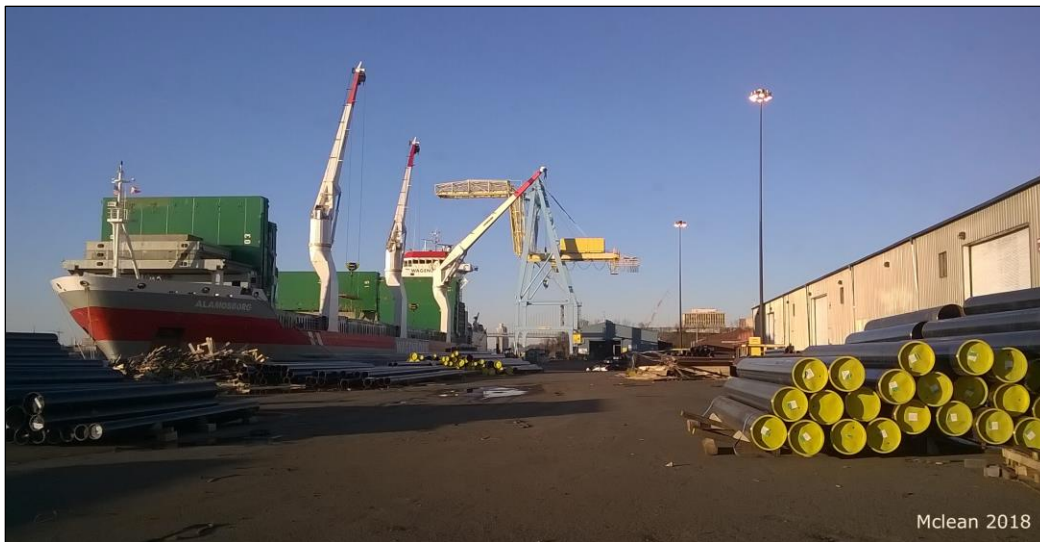
Figure 1. Ports are critical to the U.S. national economies, global trade, and national security. Photo: Port of Camden-Gloucester, N.J. (photo by Elizabeth L. Mclean, 2018).
