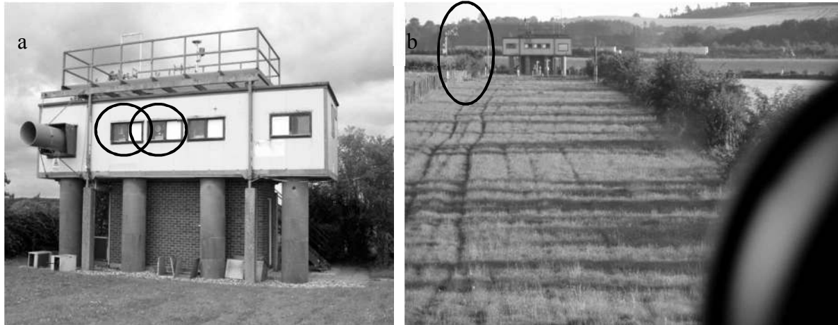
Figure 3.1 (a) K&ZLAS receiver cabin – the scintillometers are visible behind the two encircled windows. (b) View from the K&ZLAS transmitter to the receiver cabin – the eddy-covariance tower is encircled
