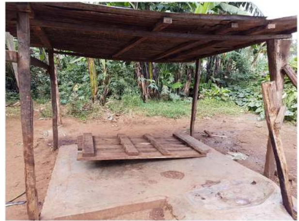
FIGURE 3 | A rural slaughter slab with a pole mounted roof and a wooden pallet. Photo: Linda Waldman.
