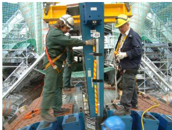
Figure 21. Installation of the barrel cryostat in the ATLAS cavern (left). The installation of the final TileCal module in the EBC calorimeter (right).
