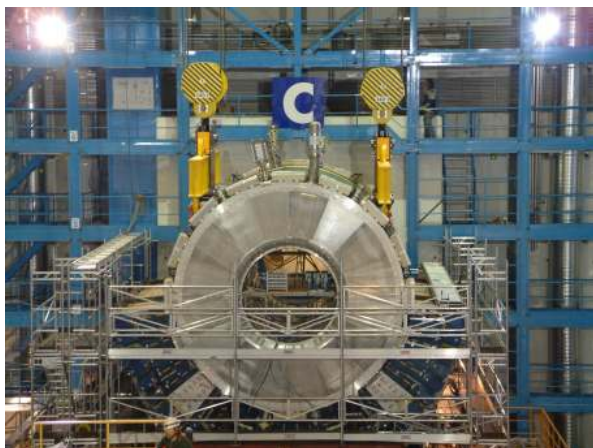
Figure 21. Installation of the barrel cryostat in the ATLAS cavern (left). The installation of the final TileCal module in the EBC calorimeter (right).
