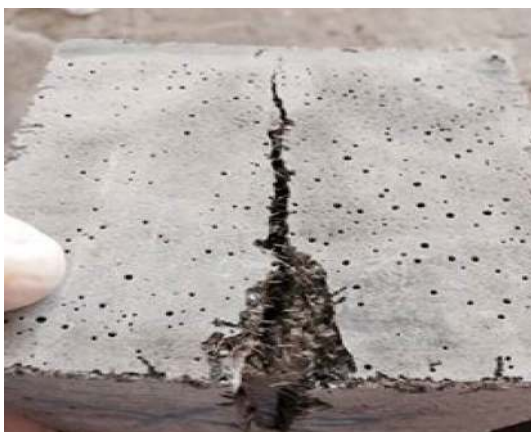
Fig. 7 Failure state in MSF reinforced UHPFRC after splitting tensile strength test
