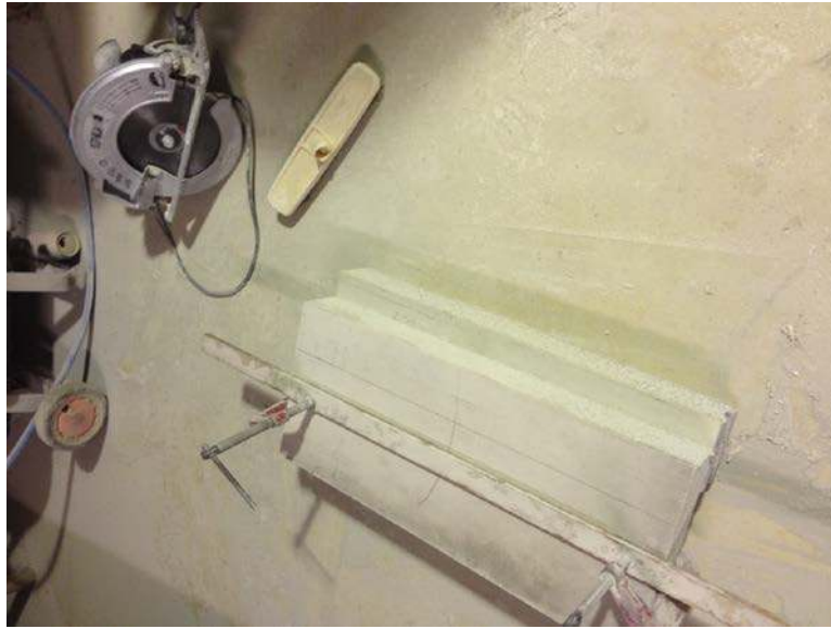
Figure 5: Measuring and cutting of full panels
