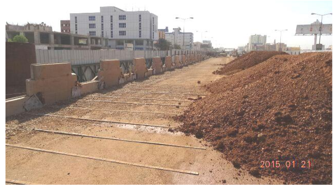
Fig. 8 The backfill material used in construction of MSE
