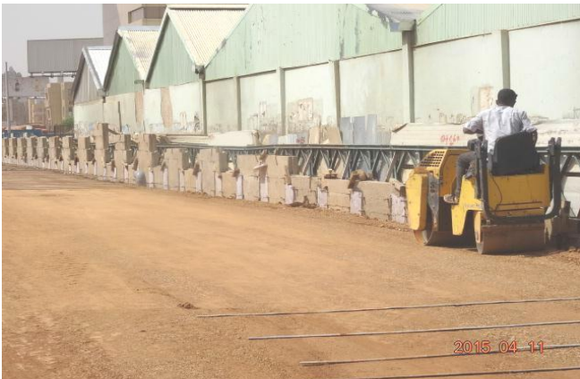
Fig. 10 Compaction by rolling of reinforced backfill soil
