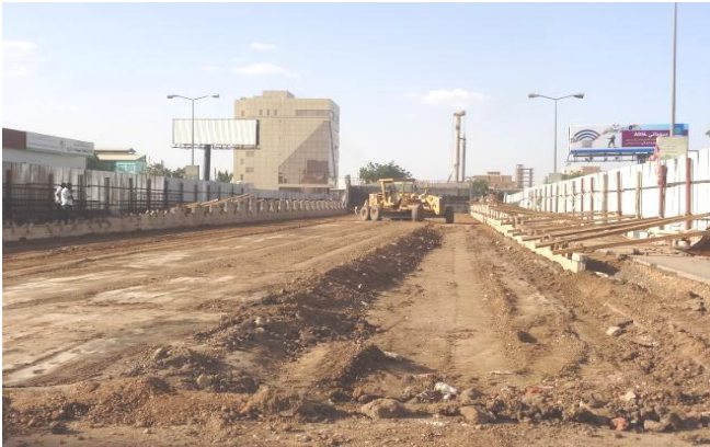
Fig. 9 Setting of the first row of precast facing panels
