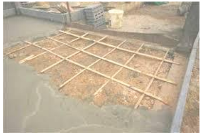
Fig. 1 Bamboo Strips used in earth construction [8]
