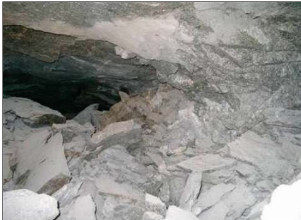
Figure 12—Up-dip side of Pillar 16
