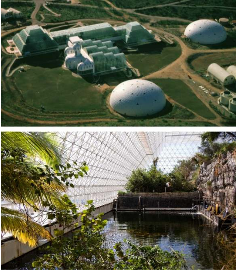
Figure B1 Biosphere 2, USA. Upper panel shows the entire biosphere facility and lower panel shows the simulated ocean ecosystem. Photos courtesy of C.T. Bannon, CDO Ranching and Development, L.P.
