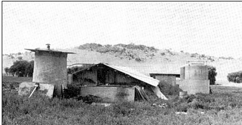
Fig. 32 Digester with storage tank in background
