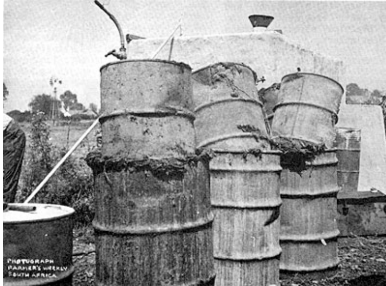
Fig. 18 Original sump digester. Upper drums have been forced up by methane
