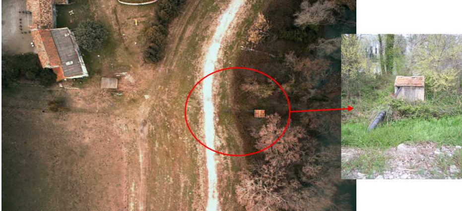
Fig. 6. 0.02 m resolution digital image acquired during the LiDAR survey. It shows a pump line through the base of a dike (source Cemagref -FUGRO)
