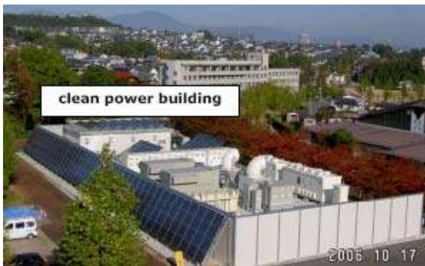
Figure 9. The Sendai Multiple SQRA Microgrid Demonstration
