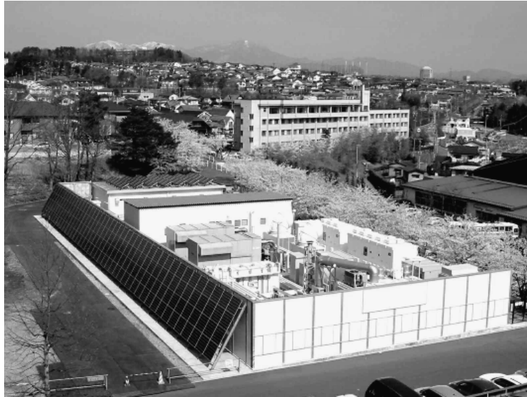
Figure 6: Sendai microgrid installation. (source: NTT Facilities)
