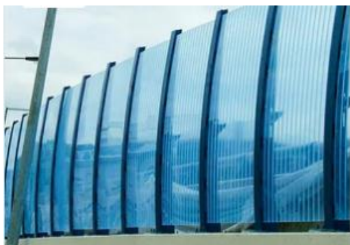
Fig. 1. Placing the screen along the motorway
