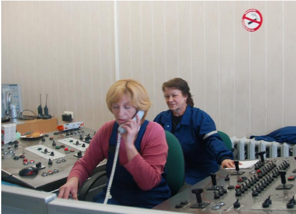
Illustration 5. The main switchboard
