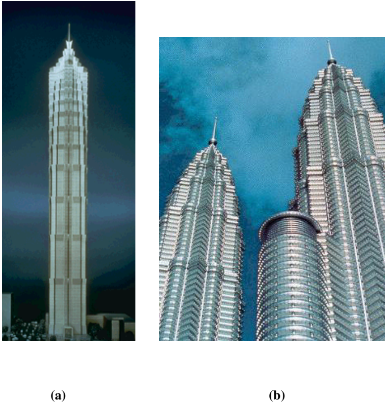
Figure 8: (a) Sketch of Jin Mao Building. (taken from Skidmore, Owings, and Merrill, LLP); (b) Photo of upper plan of Petronas Towers (taken from kiat.net)
