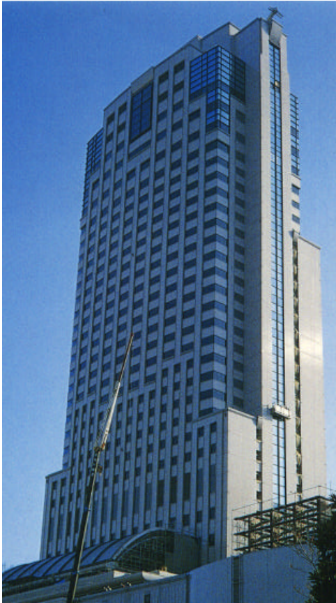
Figure 25. NTT CRED Motomashi Building (taken from Mitsubishi Heavy Industries, Ltd.)
